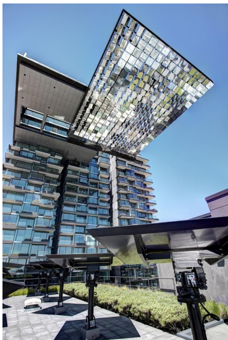
Image 7 – Heliostats targeting Reflectors
