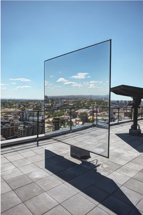
Image 9 - Heliostat Installation – One Central Park, Sydney
