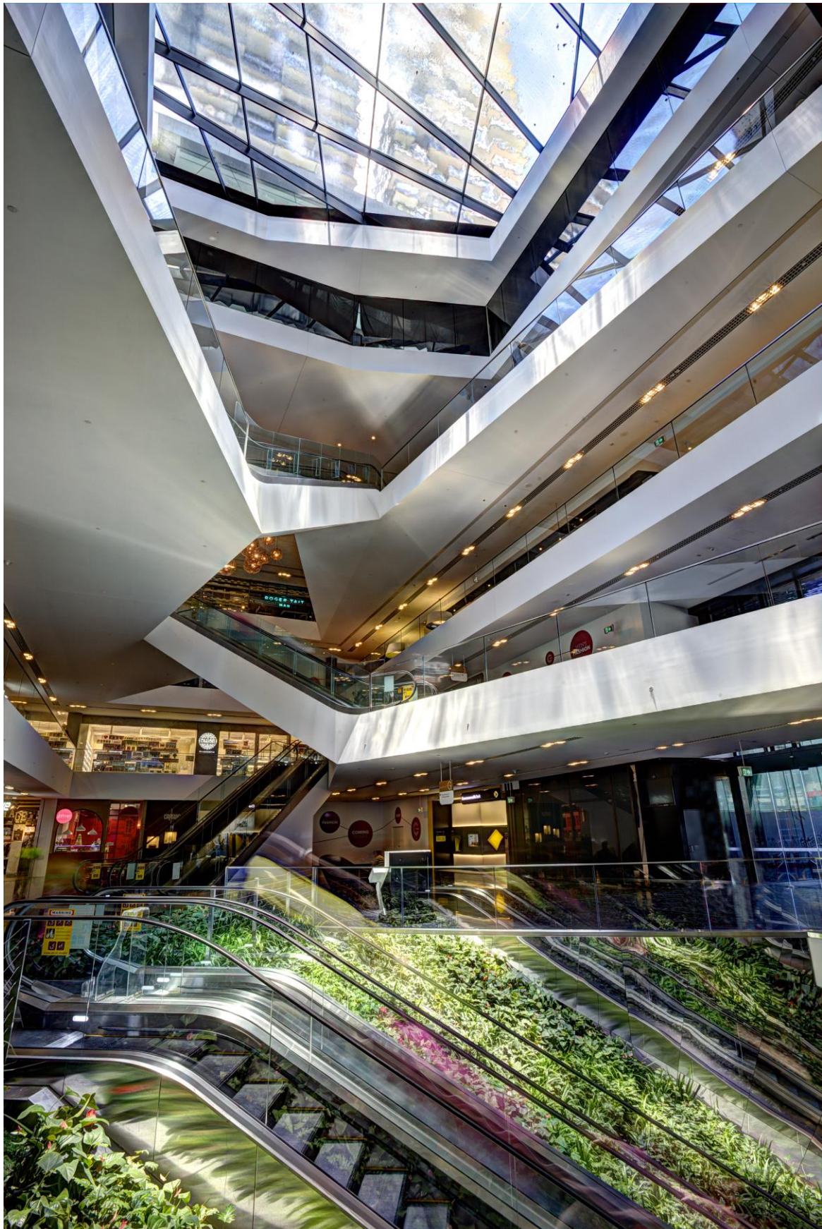
Image 12 – This is the Retail Atrium which is being lit by the Heliostat System
