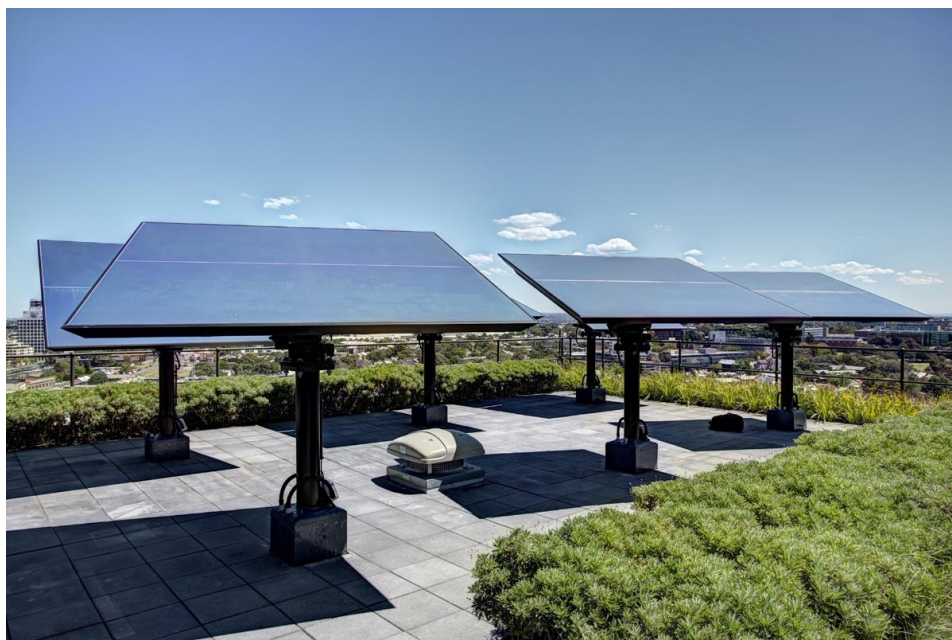
Image 11 – Heliostats tracking the sun and redirecting the sunlight
